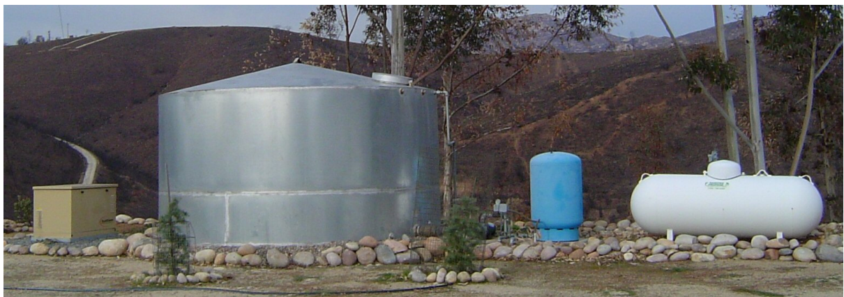
Supply and backup systems for WEEDS include from left to right a 12 kW generator, a 5000 gallon (21 k liter) storage tank, a pump, pressure tank, and propane supply.
