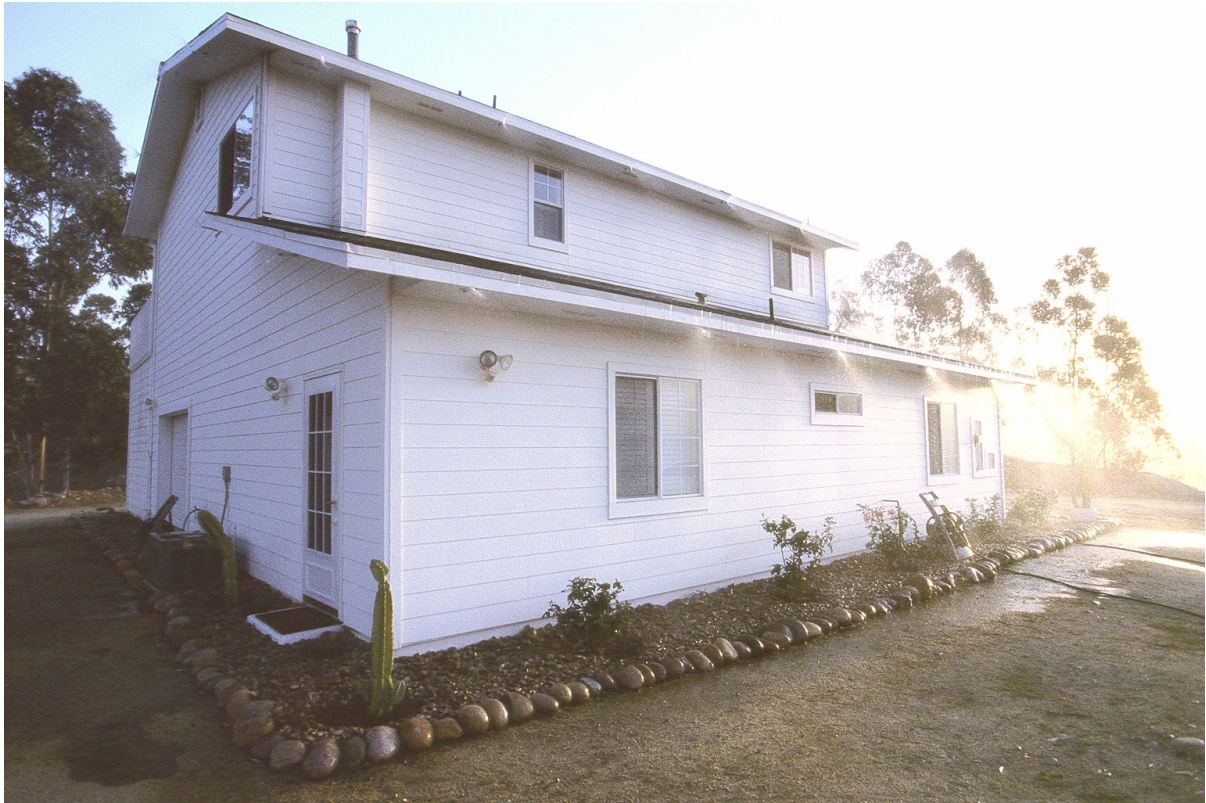
Photo of the WEEDS sprinkler system in operation. 32 nozzles delivering about 4 liters per minute each are directed away from the structure. Photo by Nanette Martin ( www.nanettemartin.com ).
